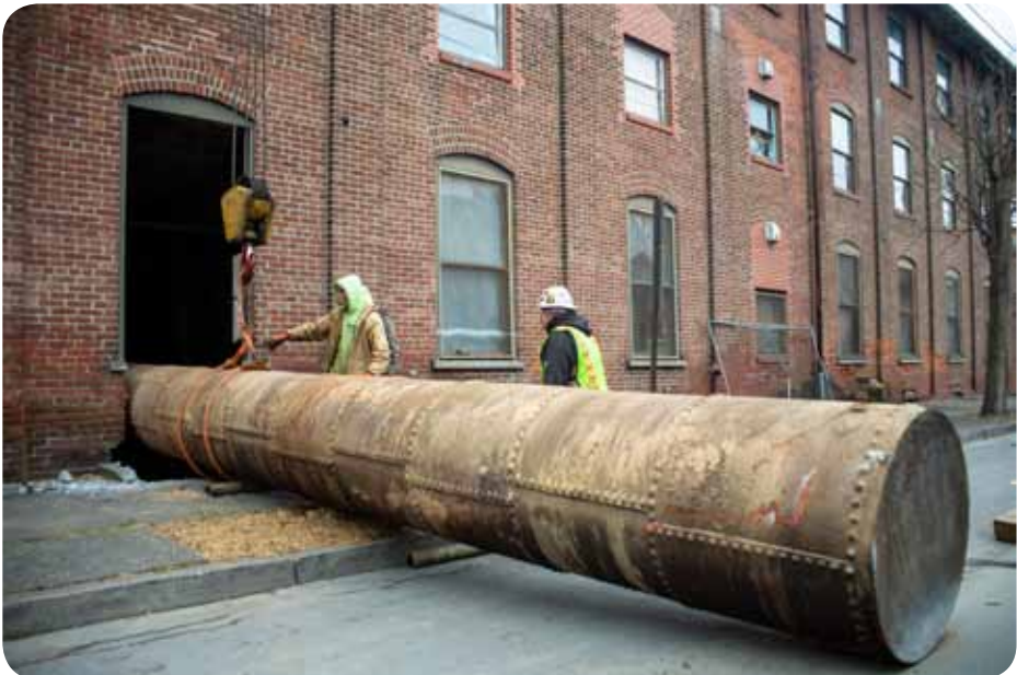
Figures 8 – 10: Photographs of the 33-inch diameter boiler being pulled through a doorway in the building made from a window opening. Photograph of the boiler in the basement as it was being lifted from its location as a water tank. Attribution for this entire set is NMIH.
