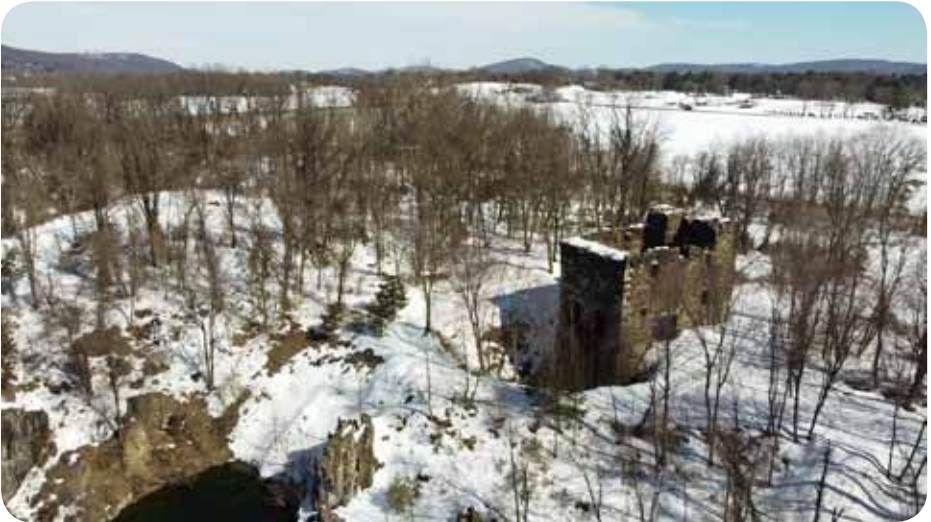
Figures 6 & 7: Engine House Ruins taken from a drone camera showing engine house, pump shaft and the water filled mine pit. Attribution is Brad Lang.
