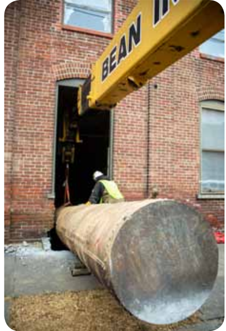
Figures 8 – 10: Photographs of the 33-inch diameter boiler being pulled through a doorway in the building made from a window opening. Photograph of the boiler in the basement as it was being lifted from its location as a water tank. Attribution for this entire set is NMIH.
