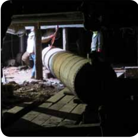
Figures 8 – 10: Photographs of the 33-inch diameter boiler being pulled through a doorway in the building made from a window opening. Photograph of the boiler in the basement as it was being lifted from its location as a water tank. Attribution for this entire set is NMIH.
