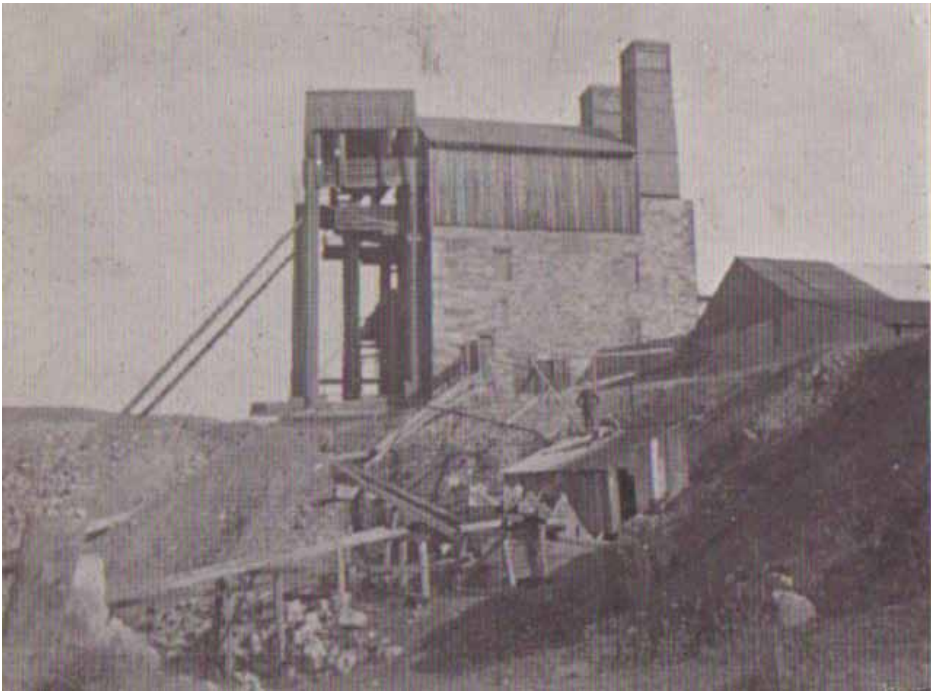
Figure 1: Postcard taken from within the Ueberroth Mine pit facing The President Engine House showing the walking beams and the pump rods. The photograph is circa 1875. Attribution is uncertain.
